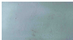
Plaster exposed for 10 years with a CRAKGON reinforced paint system.
