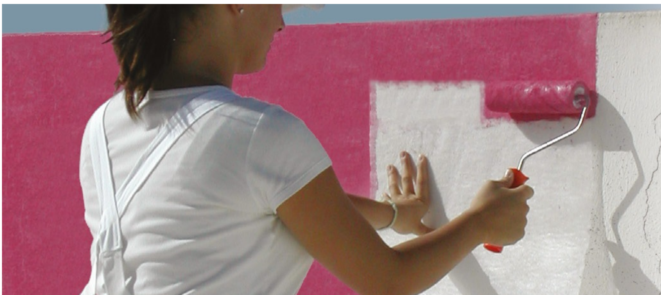
CRAKGON being applied.
